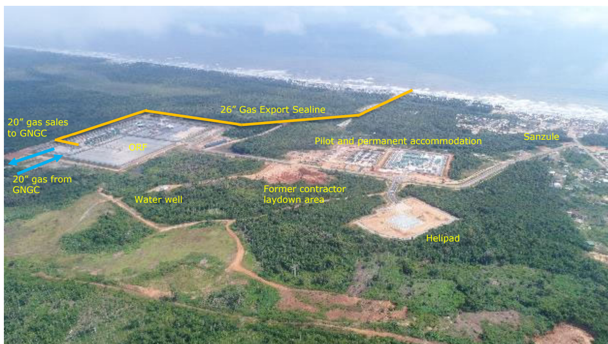
Figure 3-2: Onshore facilities (drone photo in late 2019)
