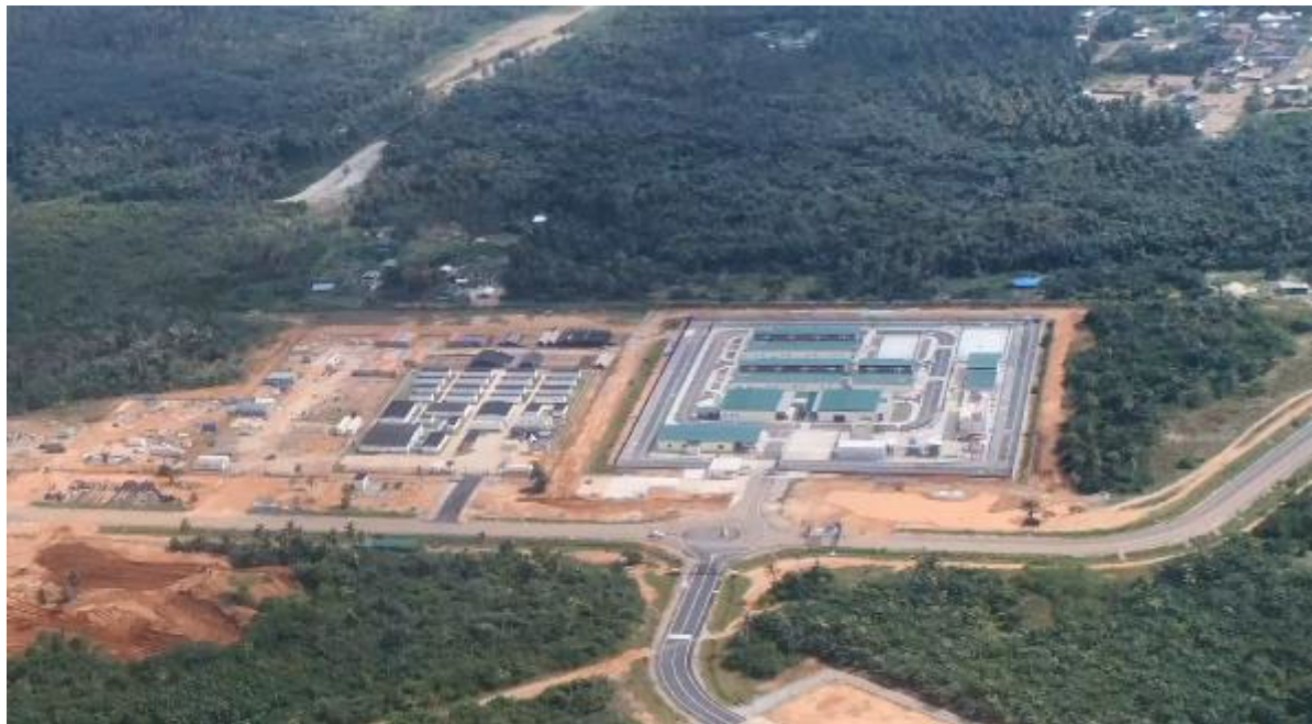
Figure 8-1: Pilot camp (left) and fully constructed Permanent Accommodation Camp (right)
