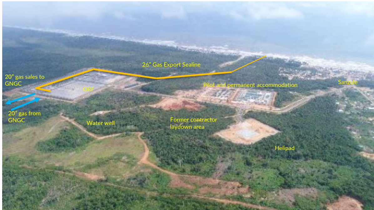
Figure 3-2: Onshore facilities (drone photo in late 2019)
