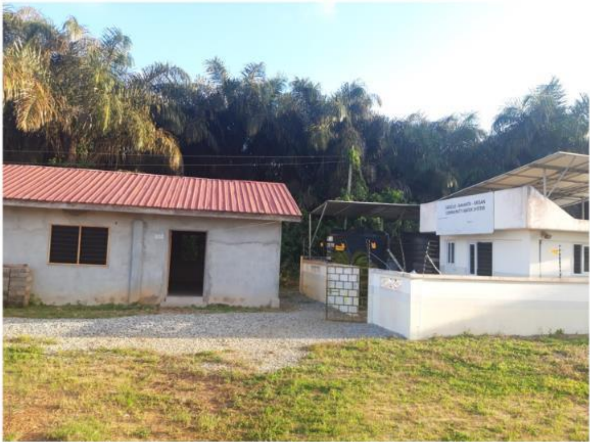
Figure 6-1: Community Water System treatment plant, with adjacent facility in construction to allow for filling of water sachets
